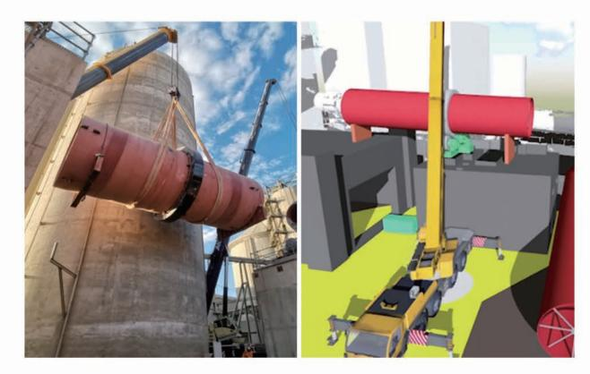
回转窑智慧吊装对比图 Contrast of intelligent hoisting of rotary kiln
