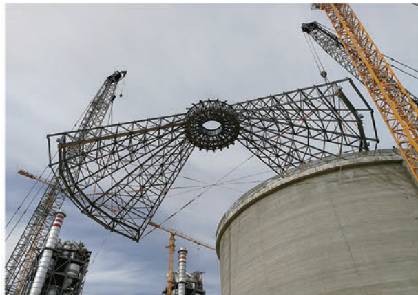
阿尔及利亚BC项目熟料库顶钢结构吊装 Hoisting method of the clinker silo roof steel structure of BC project in Algeria
