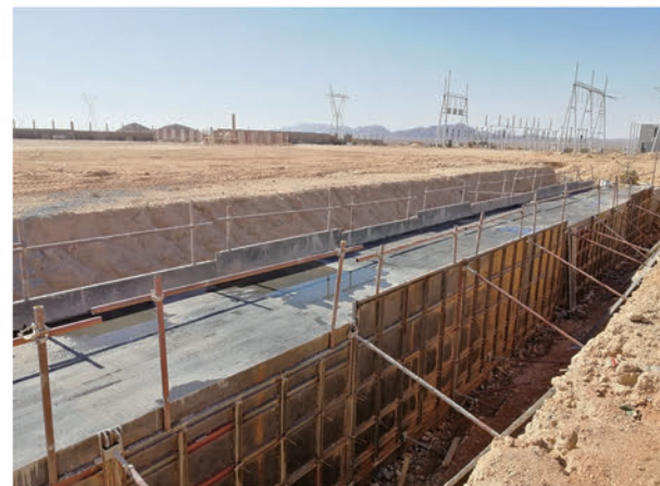
阿尔及利亚BECHAR项目电缆廊道内外侧定型模板安装 Installation of stereotyped formwork inside and outside cableway of BECHAR project in Algeria
